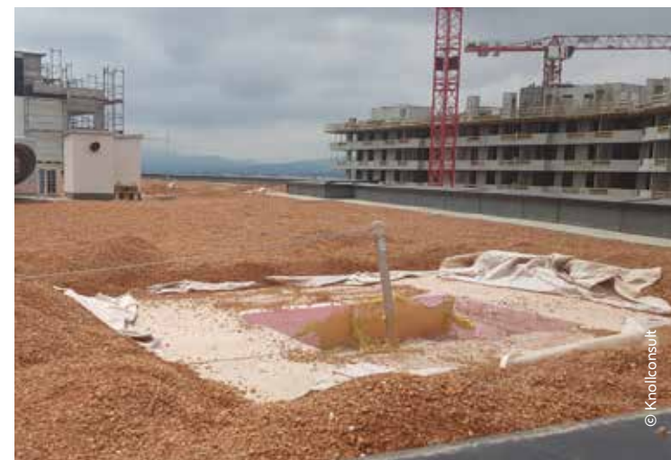
Modeling of the substrate for extensive greening
