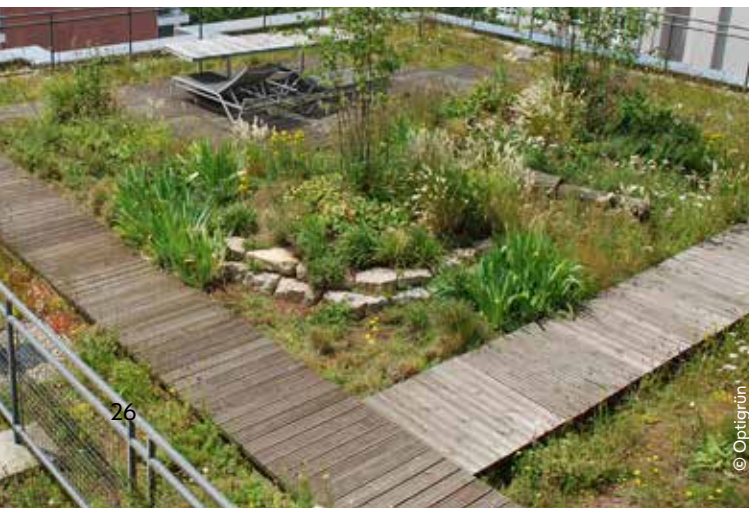
Extensive green roof: example of a „natural roof“
